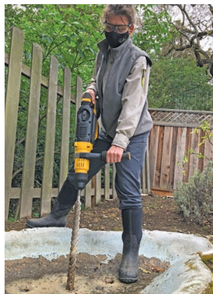
Vector Control Technician Kim drills holes in an old decorative water feature at the request of a resident to help reduce water where mosquitoes can breed.
